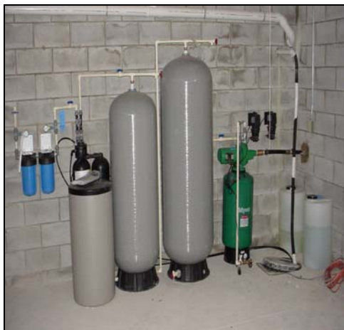
Typical Home Surface Water System
